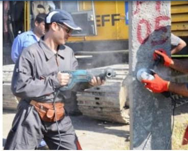
Pile preparation before fixing sensors
