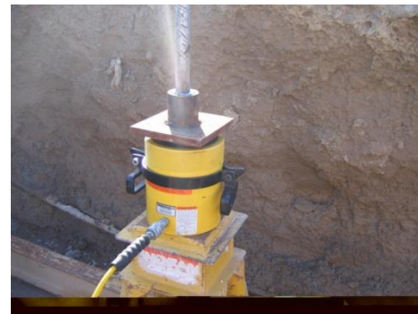
Static tension test of micropile
